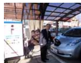
EV quick-charging facilities
